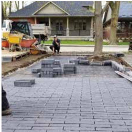
"You stage pavers throughout the job without damaging your prep work. Big time savings!"
